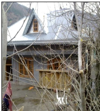
Figure 2: modern house with a Aluminum sheet
