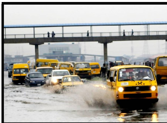
Figure 2: Flooded Road in Lagos
