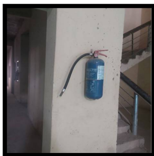
Figure 4: Image Showing Fire Extinguisher Close to the Fire Escape Staircase Source: Author's Fieldwork, 2022
