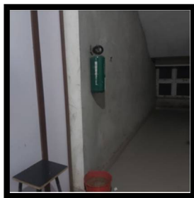
Figure 3: Image Showing Sand Bucket and Fire Extinguisher Positioned in Front of a Studio Source: Author's Fieldwork, 2022
