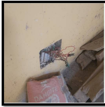
Figure 10: Image Showing One of the Many Exposed Sockets in the Building Source: Author's Fieldwork, 2022
