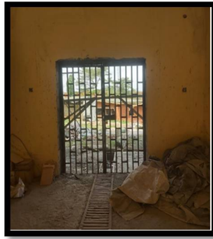
Figure 7: Images Showing Blocked Exit Points in the Building Source: Author's Fieldwork, 2022
