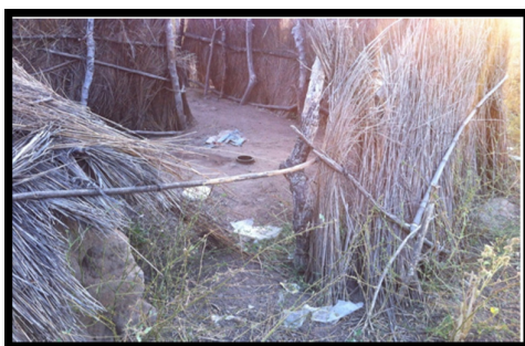
Figure 5: A Toilet with Walls Made of Grass in a Household in Djouroum, Rey Bouba Source: Fieldwork
