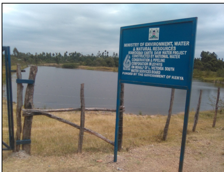
Figure 4: Kamogiboi Dam Site
