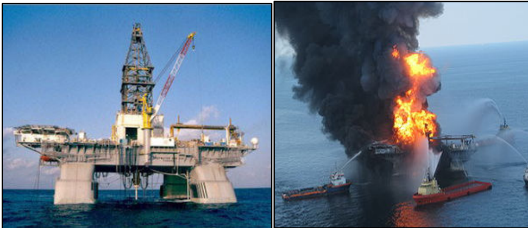
Figure 2, and Figure 3: Showing the Macondo flat form before and after the blowout
