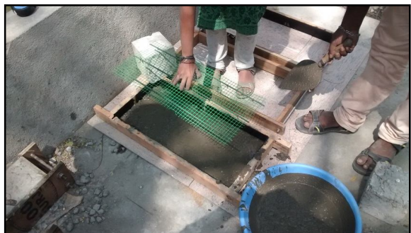
Figure 10: Laying of Mesh with Skeletal Steel
