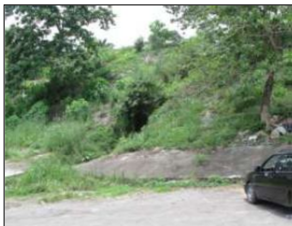
Figure 7b Left wing of the successful slope-stabilization works at the Marina in Calabar. (Photo credit: Ukorebi, U. A.)
