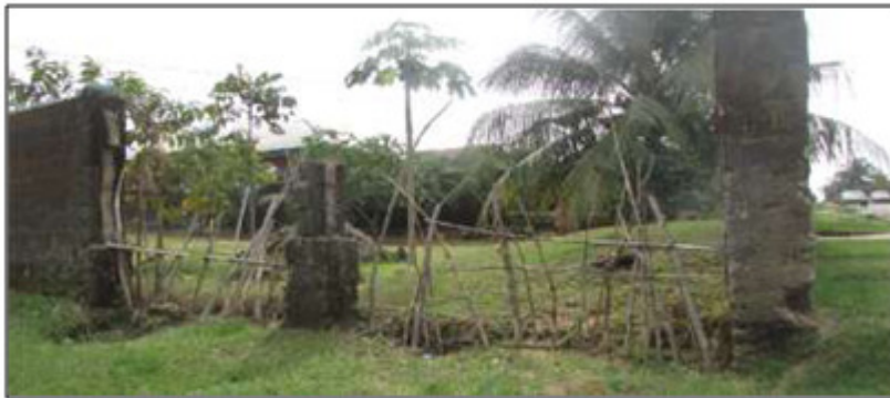
Figure 3a: By reason of the dramatic increases in volumes of stormwater that followed rising imperviousness, random overflow of stormwater occurred frequently in the territory. The two openings in the fence of this compound represent the portions that were pulled down during the rainy season of 2014; they have not been repaired ever since.
