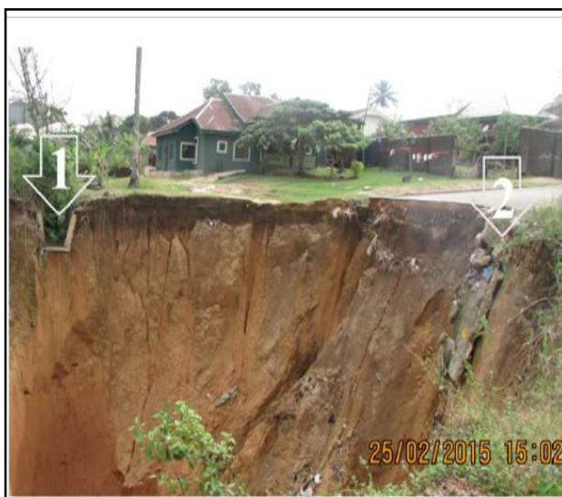
Figure 4b: The termination of the paved road and concrete drains at the valley's edge in Sector-A of the study area
