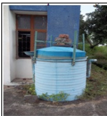
Figure 4: Biogas Digester
