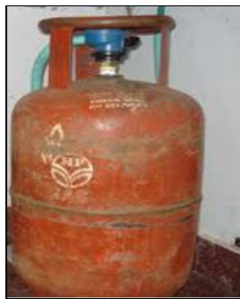
Figure 5: showing LPG cylinder with Regulator and hose pipe
