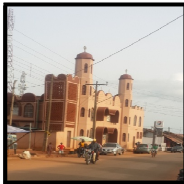
Figure 5: Central Mosque Completed between 20-30years fairly affected by weather Source: Authors Field Photograph (2017)
