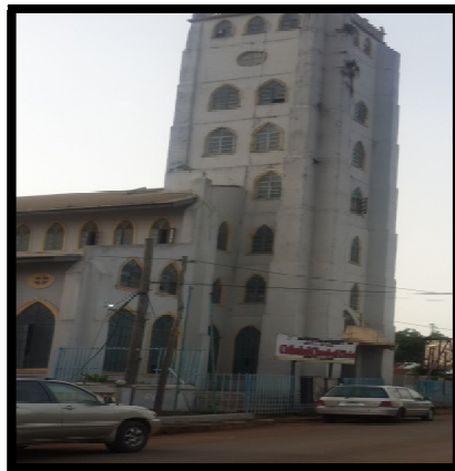
Figure 4: Cathedral Church Ona Ola Road Completed for Over 50 Years Enjoys Regular Maintenance Source: Authors Field
