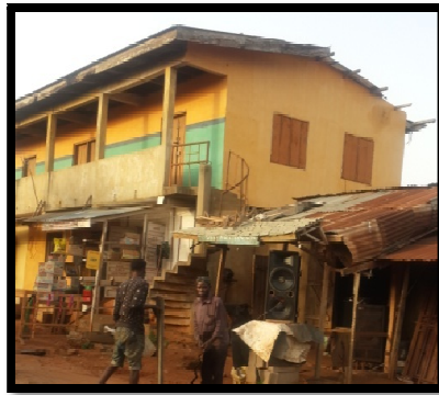
Figure 3: Commercial Building at Orita Oja Odan Road Completed for Over 20 Years fairly affected by Weather Source: Authors Field Photograph 2017
