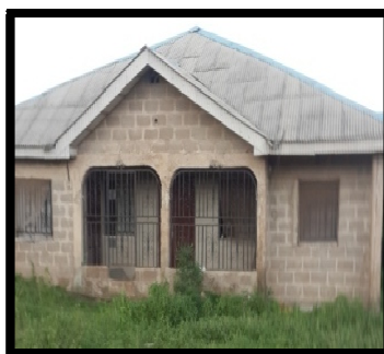
Figure 10: Residential Building with Unplastered Block Wall in Use for Less Than 10 Years at Express Road
