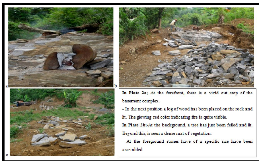
Figure 6: Rudimentary Quarrying Technique Behind College Vogt May, 2012
