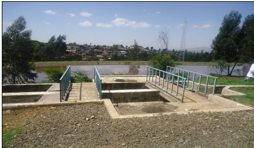
Figure 2: waste water treatment plant 2014 G C
