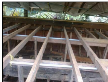
Figure 6 : Deck Beams
