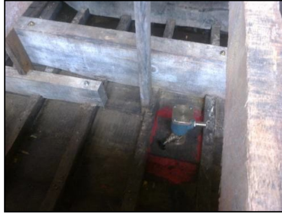
Figure 3 : Hull Bottom In way of Engine Girder
