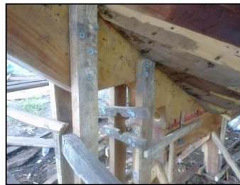
Figure 5: Aft End Construction
