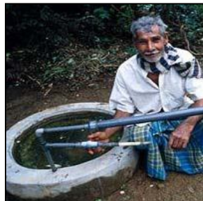
Figure III : Pipes for passage of biogas
