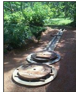
Figure II: Covered tank or digester
