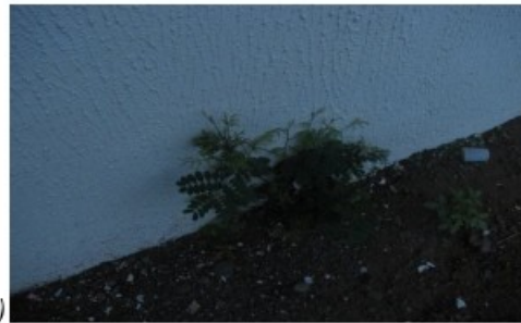
Figure 3 a and b: L. leucocephala having its root into the foundation of a building. Figure 3a is the Stump of L. leucocephala deep into the foundation.
