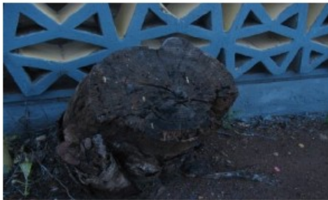
Figure 3 a and b: L. leucocephala having its root into the foundation of a building. Figure 3a is the Stump of L. leucocephala deep into the foundation.
