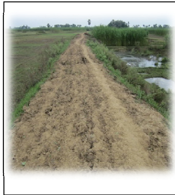
Figure 2: New Constructed Road
