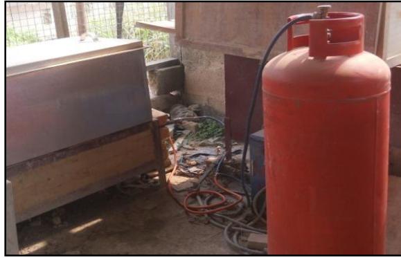
Figure 9: Gas fired bamboo boiler for preservation
