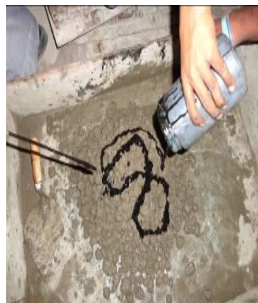
Figure 5: Mixing Of Epoxy To The Cement Concrete
