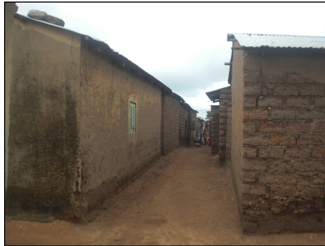
Plate 1: Traditional Houses built with mud bricks (no cement and not baked) at Nakore (Picture taken on 26 th July, 2013) Source: Author
