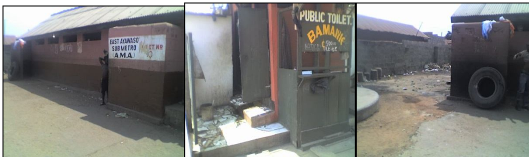
Some public toilet facilities in the Nima community
