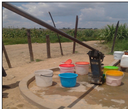
Figure 1: Community Borehole in Hopley Suburb Source: Fieldwork (2015)
