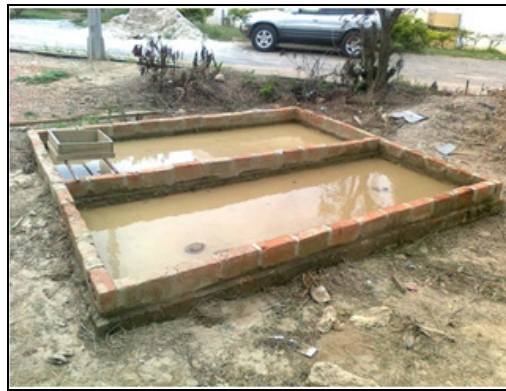
Figure 14: The soaked clay in the pit.
