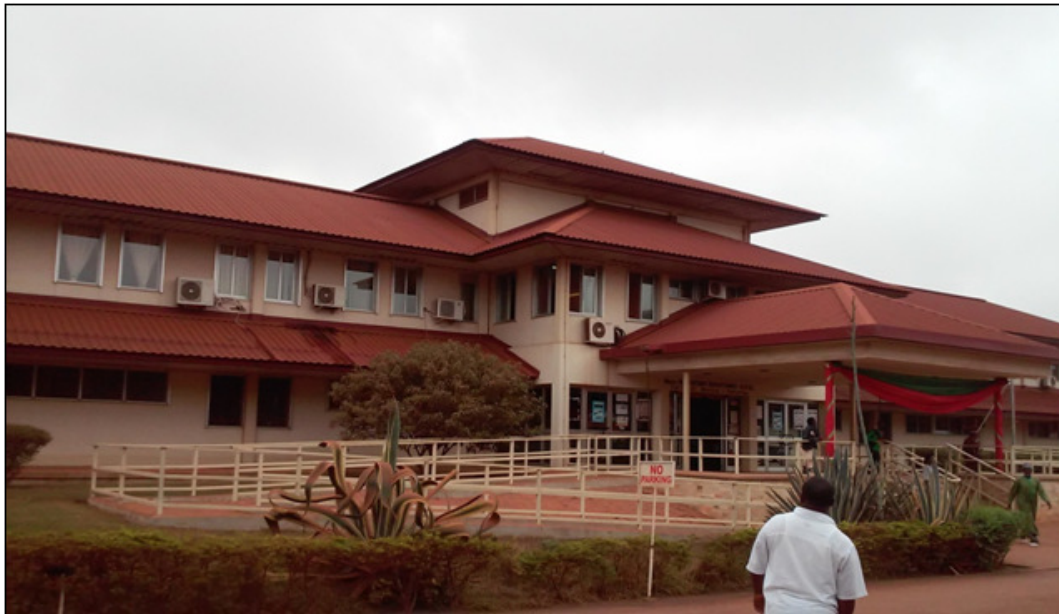
Figure 6: Brong Ahafo Regional hospital building, Sunyani
