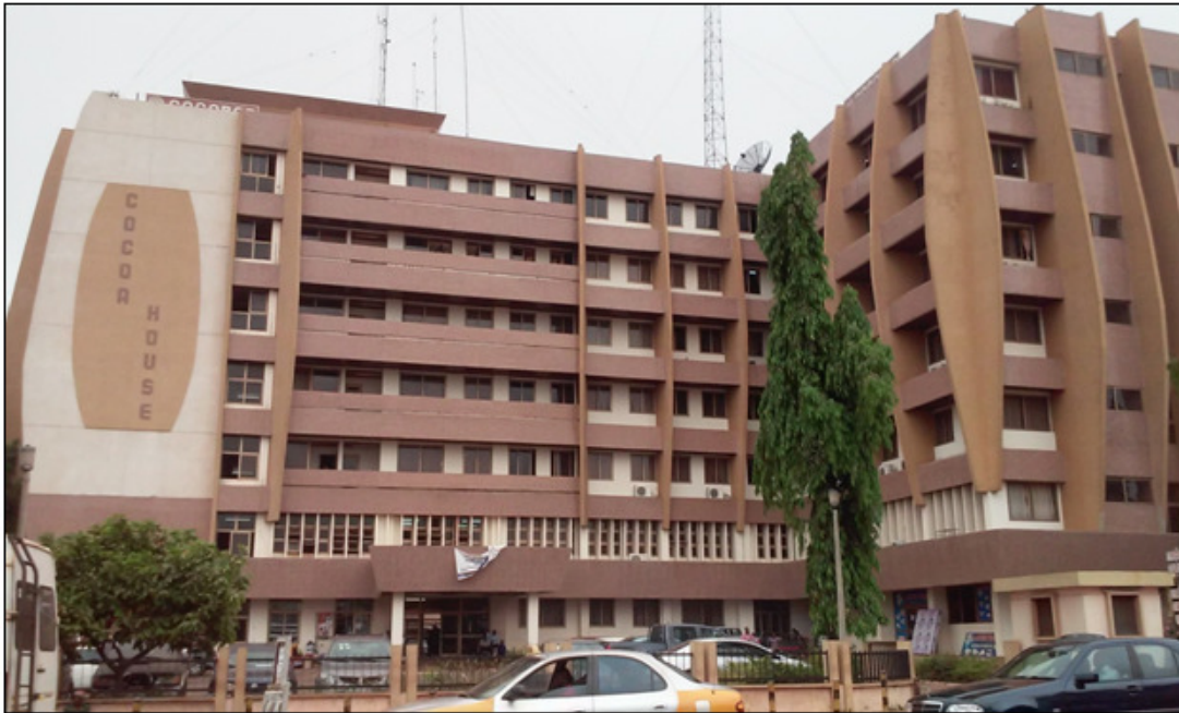
Figure 3: Six storey cocoa house building
