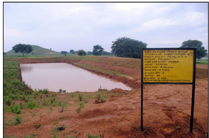
Figure 5: Water harvesting structure in Pastipada
