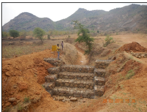
Figure 6: Loose Boulder Check Dam
