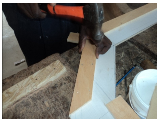
Figure 5: Constructing a footing for the stand
