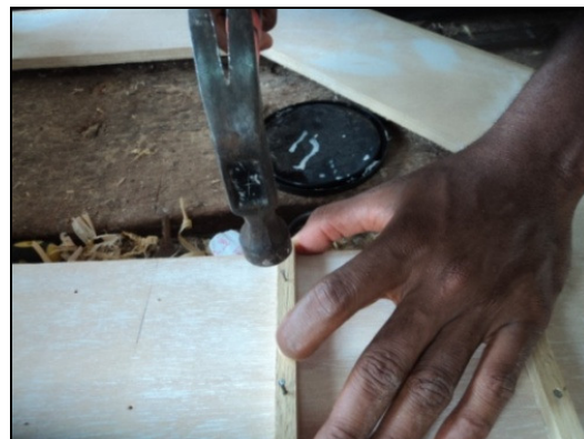
Figure 8: Nailing a stopper to the footing of the vertical support
