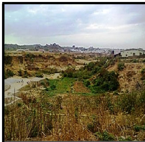
Figure 10: The reality of Erosion Menace on site Source: Researchers' Field Work, 2018
