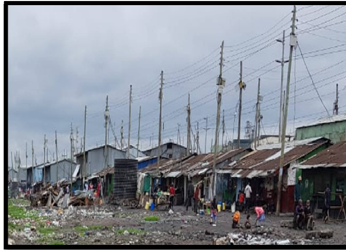
Figure 4: Image Showing Rusted Iron Sheets In Mukuru Informal Settlements Source: Author (2019)
