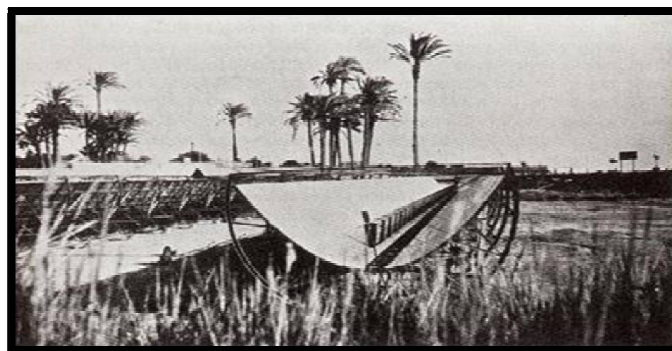
Figure 1: Shuman-Boys Solar Power Plant, Egypt
