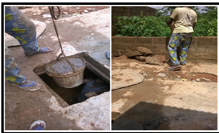
Figure 7: Process of Faecal Sludge Emptying (Manual Pit Emptying)
