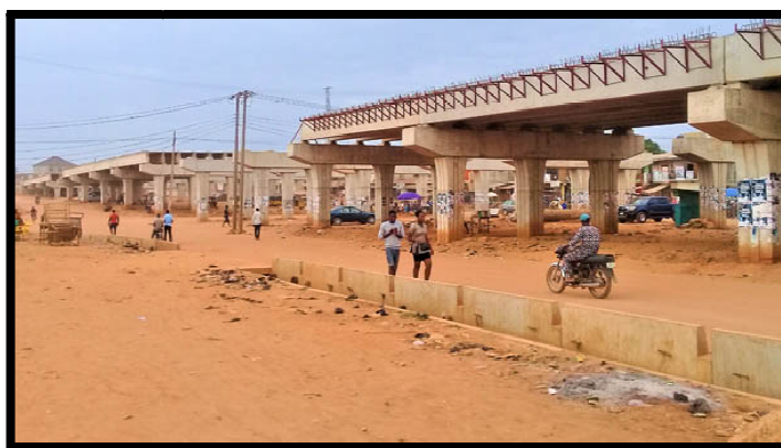
Figure 1: Ijoko Bridge under Construction
