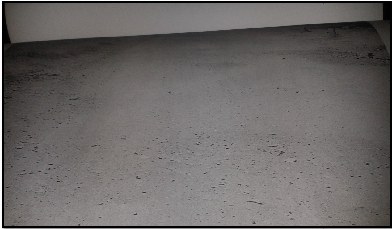
Figure 15: Pfura Road Patching Project
