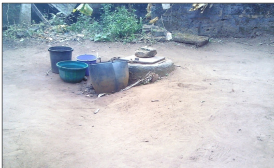
Figure 7: Underground water tanks used in storing rain water collected in an unsanitary manner
