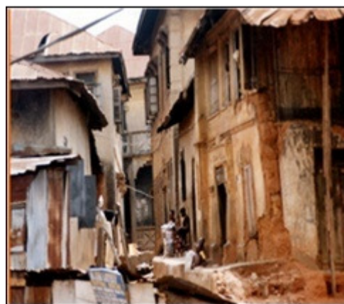
Figure 2: Accessibility and roof condition in the area
