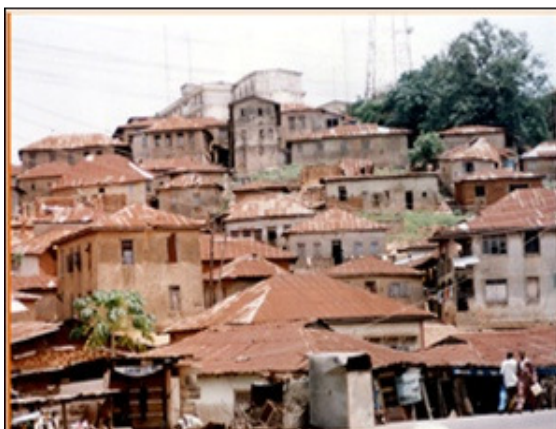
Figure 1: physical patterns and roof condition
