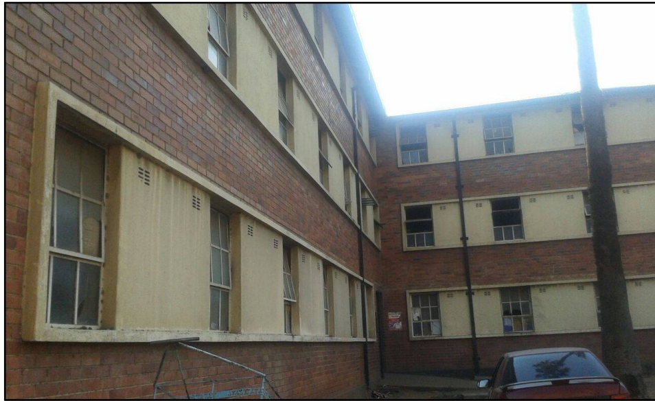
Figure 3: Sidojiwe Flat in Makokoba Source: Field Survey (2016)
