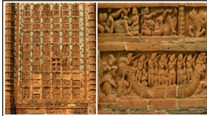
Figure 5: Multiple terracotta reliefs of 17 th century https://physicsswagata.wordpress.com/2015/06/26/poetry-in-brick-and-clay-part-2/ , accessed on 26/03/2016
