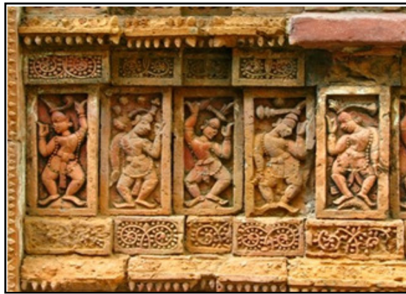
Figure 7: Terracotta ornamentation on the wall of Brick temple of Bengal http://g4.img-dpreview.com/65D02B5B92304A58844C15658E8919EA.jpg accessed on 3/4/2016
