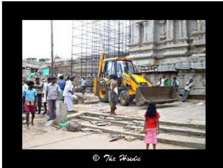
Figure 11: Work Going On
