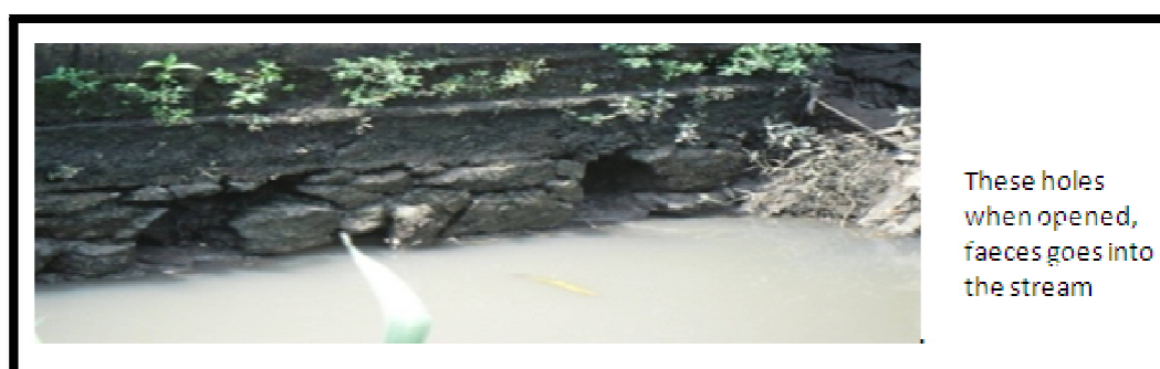
Figure 1: Perforated Pit Toilets and Septic to Water in Besseke and Bessengue, Douala (Respectively) Source: Kah Evansfigure15
