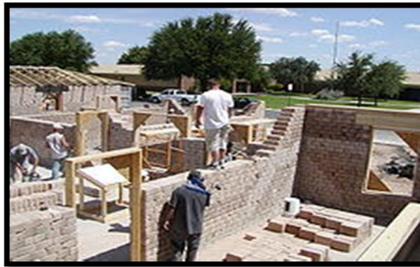
Figure 26: An Ongoing Construction Using Compressed Earth Bricks
