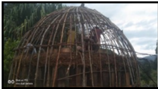
Figure 3: Honai Roof Frame (Photo: Jeninus Wenda, 21 January 2024)
